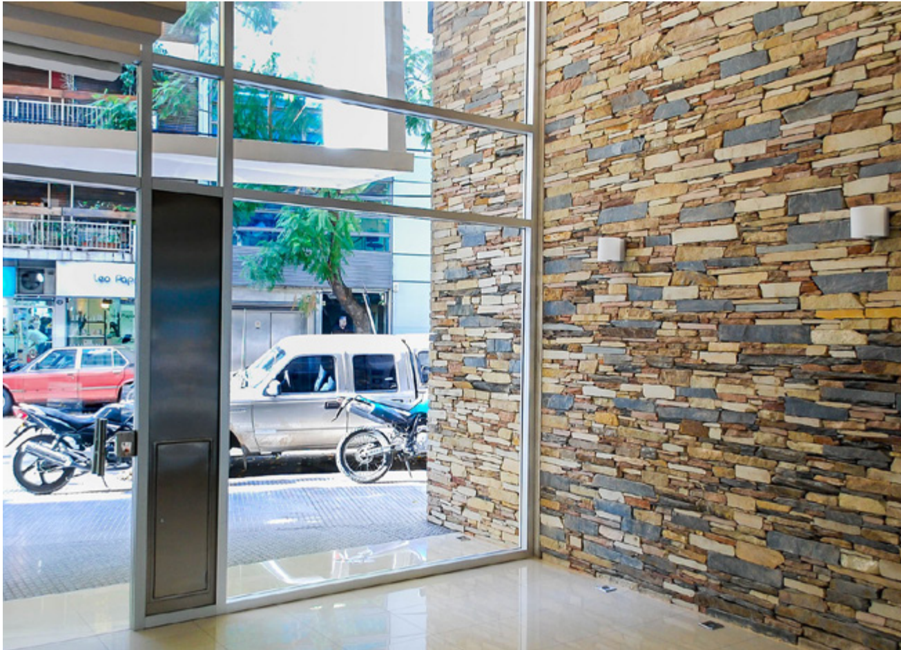
Entrance Hall Featuring Natural Stone Finishes Modelle Ocampo Building, Buenos Aires, Argentina
