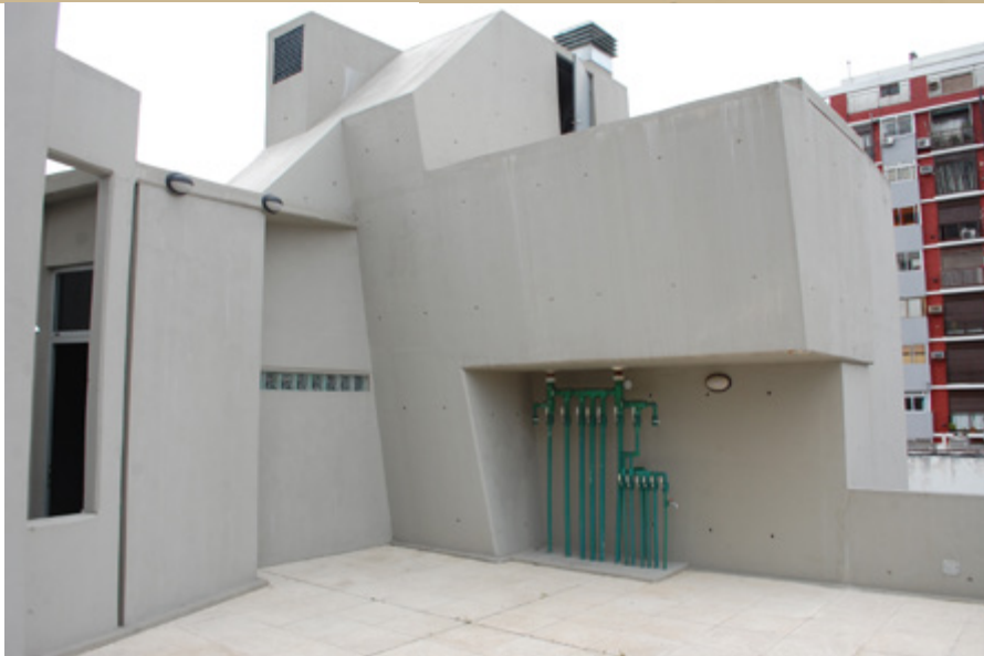
Plan, section, and 3D sketch. Finished result below. Modelle Plaza Building, Buenos Aires, Argentina
